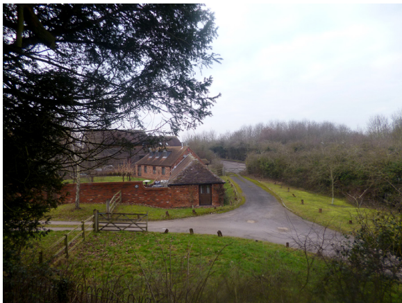
Rebuilt red brick farm buildings
