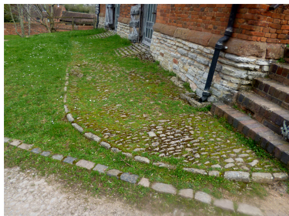
Historic surface at stable building
