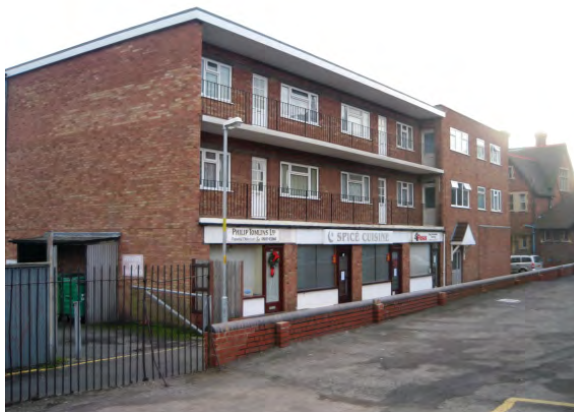
A negative impact, Nos.37-43 Bromyard Terrace.
