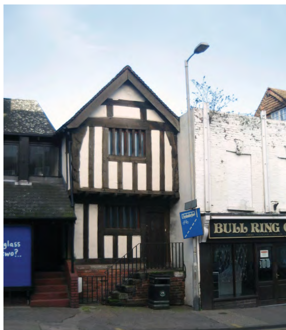
No.6 St Johns, rebuilt framing to front but older fabric is behind.
