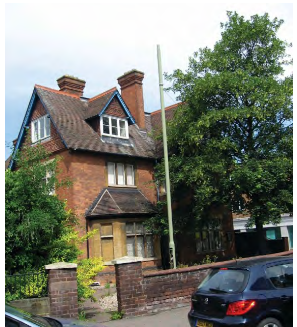
Former vicarage and the lime tree.
