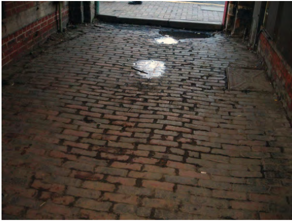
Old brick paving to alley – No.31 St. John's.
