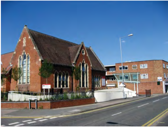
Ramp at the library – a striking colour.
