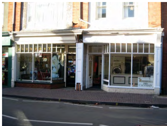
Pair of shop-fronts a century old.
