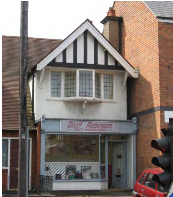
No.27 Bransford Road, in a row recommended for inclusion in future
