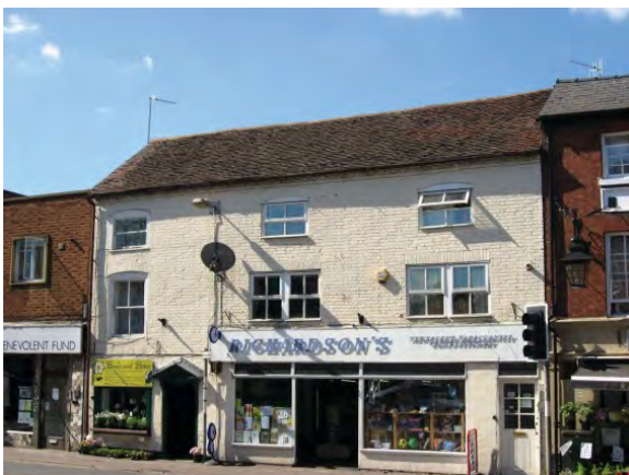
Locally listed – once a terrace of three houses, Nos.26-28 St Johns.
