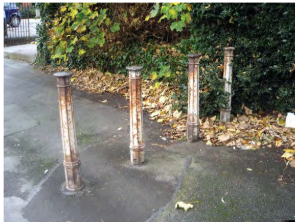
Bollards across Bromyard Terrace.
