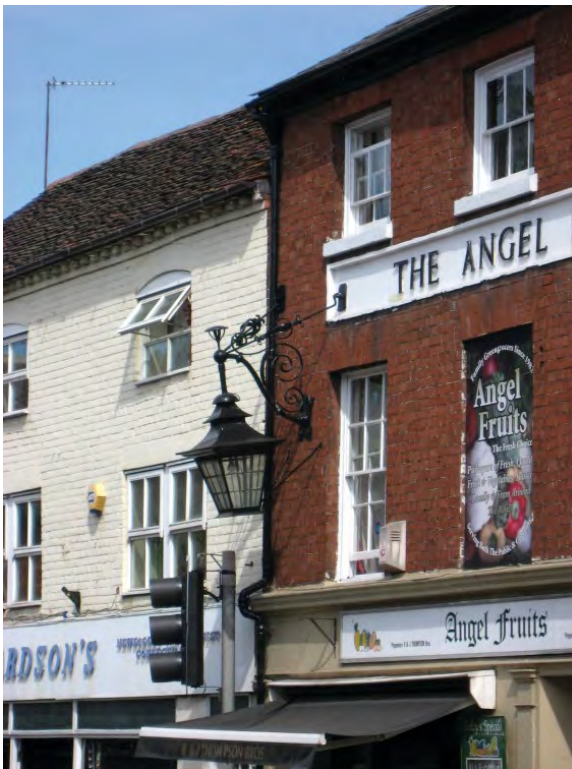
Lantern (relocated away from the traffic).
