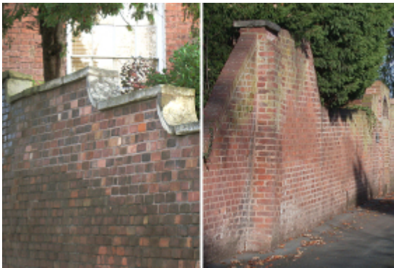
Garden walls with stone or brick copings - Rose Hill and Rose Bank.
