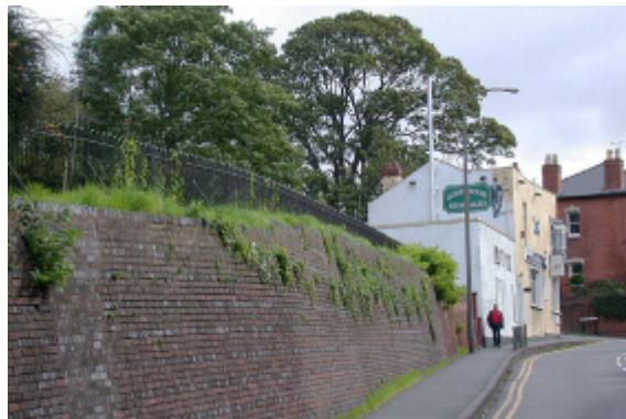
London Road cut into the hillside
