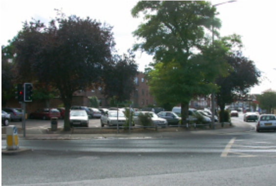
The car park makes an unsightly gap in Sidbury.
