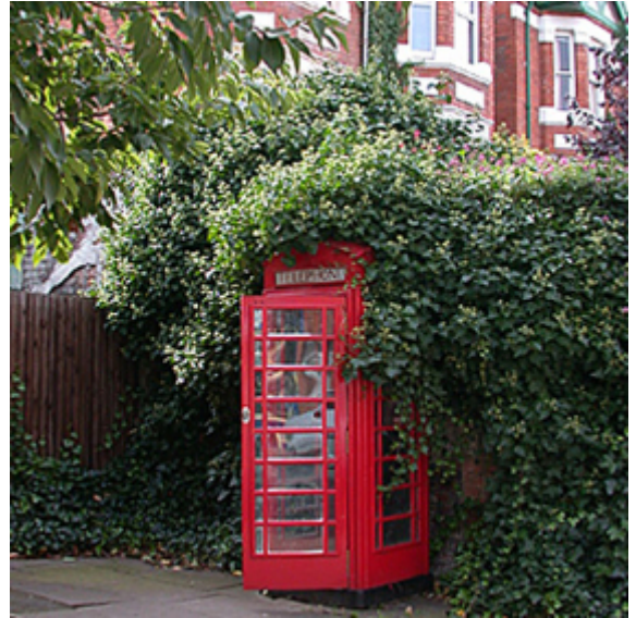
A listed structure, telephone kiosk in Bath Road
