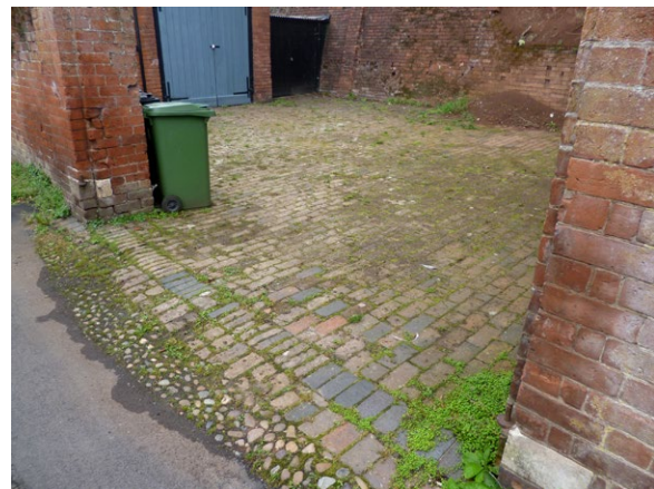
Historic Surfaces, Lark Hill
