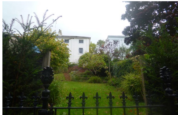
Detached 'villa' house
