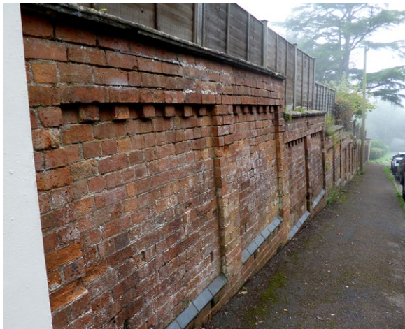
Stepped brick wall with good detail, Lark Hill Road
