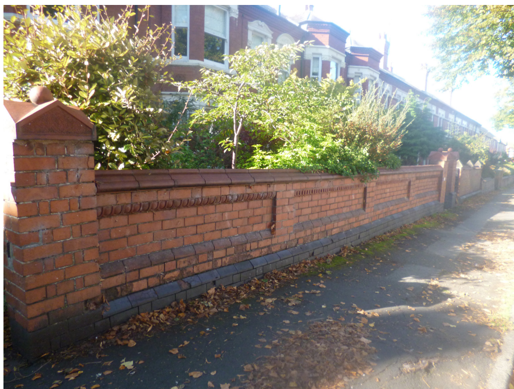
One of a variety of historic garden walls and boundary treatments
