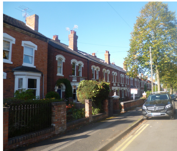
Terraced Housing, front gardens and a tree-lined avenue
