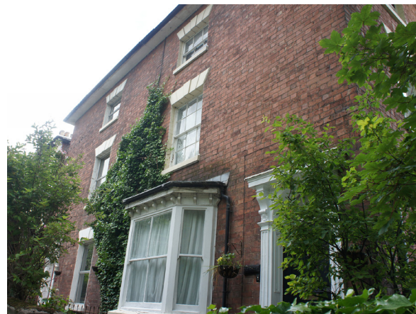
Bow window at 58 Bath Road
