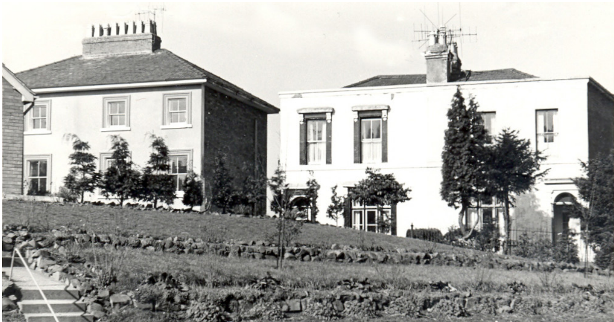
The open aspect of Field Terrace until trees were planted following the construction of 70-88 Bath Road in the mid-20th century
