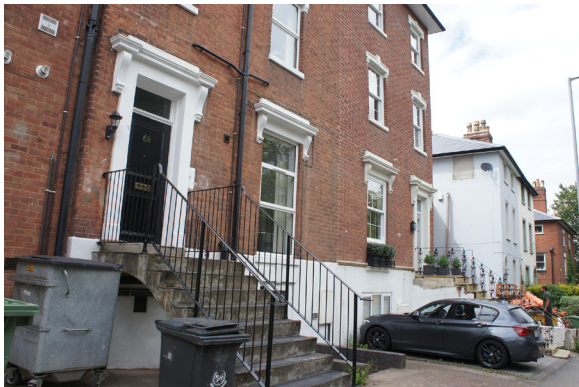
58-68 Bath Road. 66 and 68 are raised by steps
