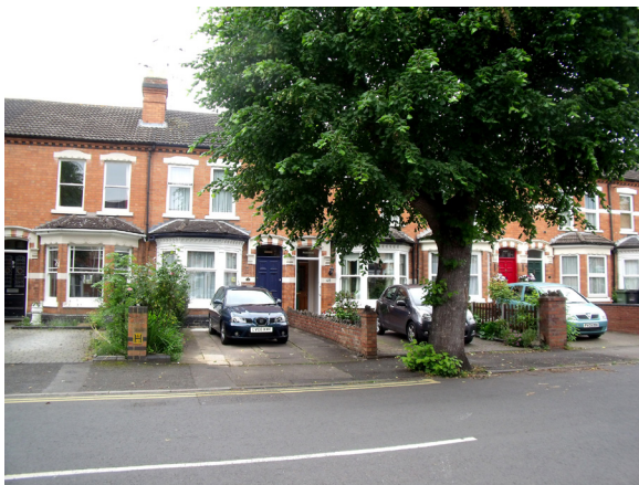
Negatively, in some instances walls have been removed to provide parking
