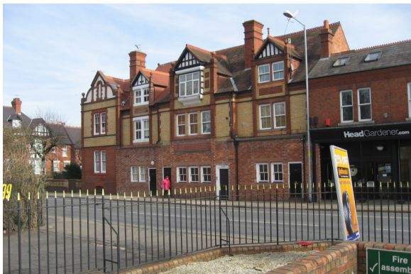
Large scale buildings on Barbourne Road
