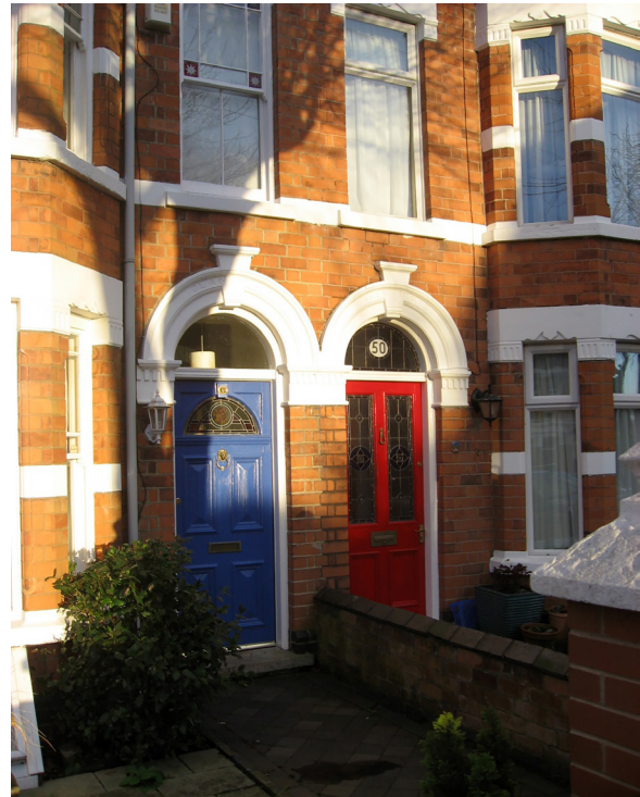
Historic architectural detailing survives alongside the negative introduction of PVC windows
