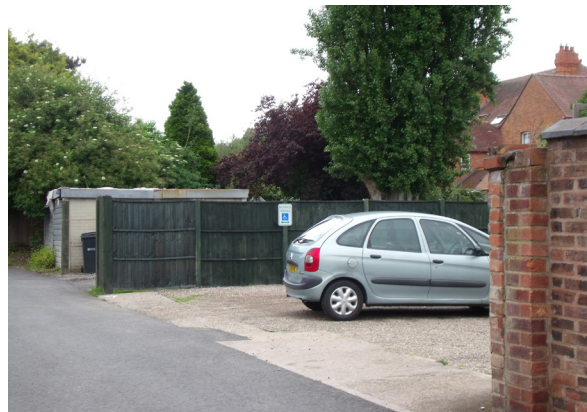
Negatively, in some instances walls have been removed to provide parking
