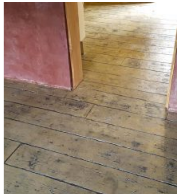
The floor is concrete, with an antique wood effect pattern, and sealed to give a gloss finish.
