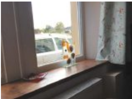
The window sills are made of hardwood.
