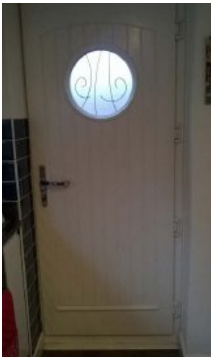
Flood resilient doors have been installed.
