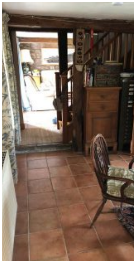
Floor is tiled, enabling them to just sweep the flood water out of the doors.
