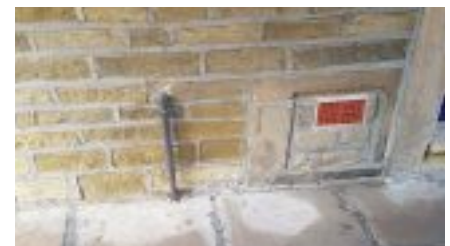
Walls were repointed and coated with a water proof spray and self-closing airbricks fitted.
