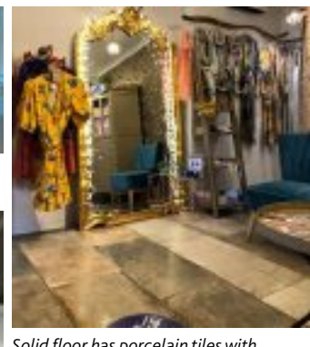
Solid floor has porcelain tiles with waterproof grout and adhesive.
