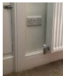
Raised plug sockets and non- return valves to washing machine and dishwasher.
