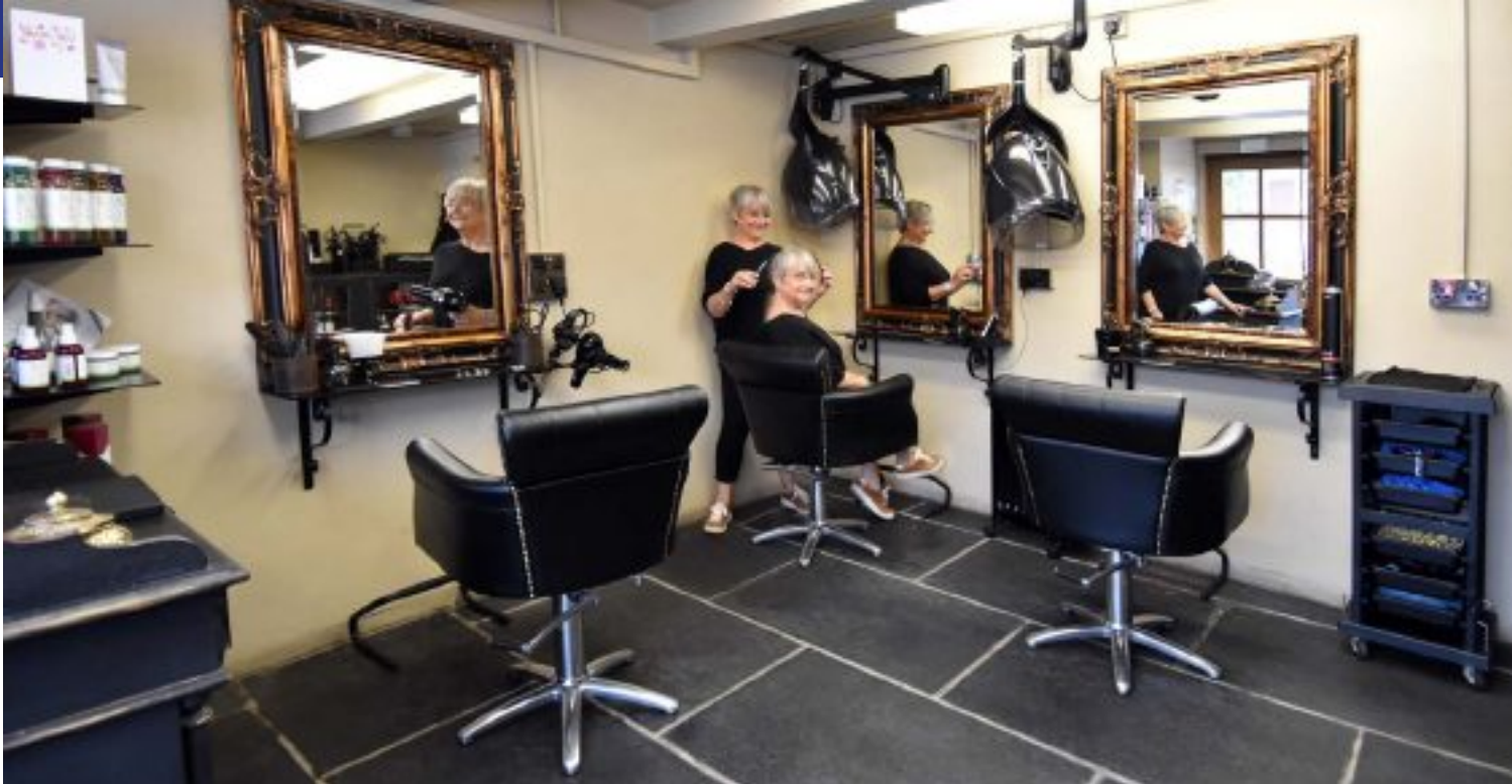
Stone flagged floor and the walls have a plastic membrane from floor to ceiling, with cement render over the top.
