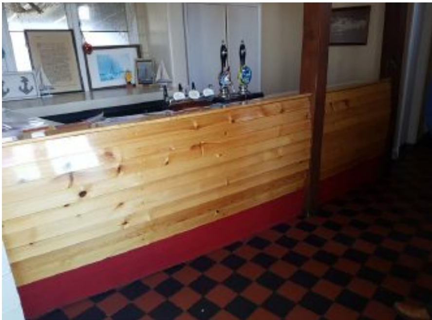
The bar is made of marine ply.
