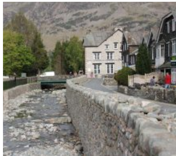
Newly upgraded Environment Agency defences.
