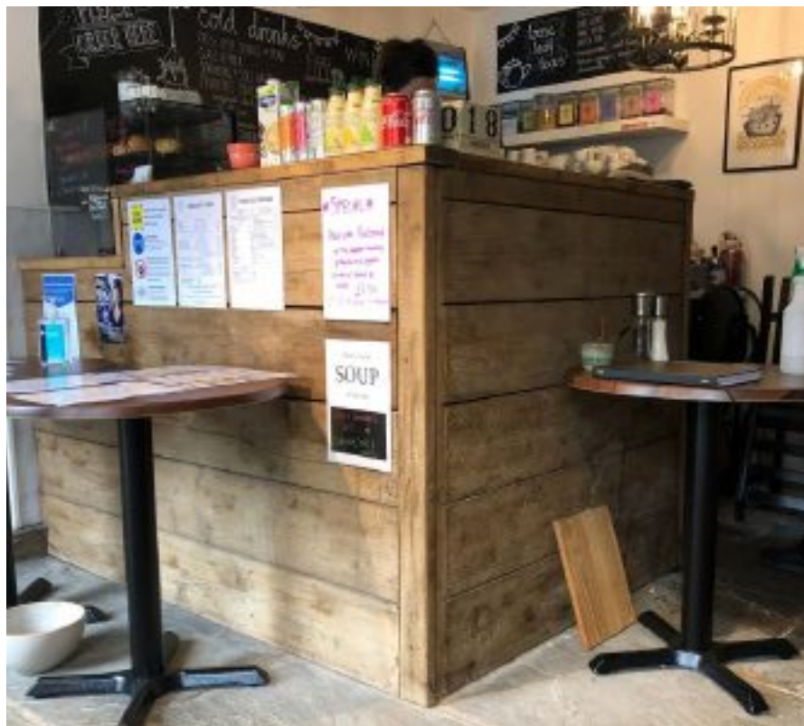
Main counter made of varnished scaffolding planks.
