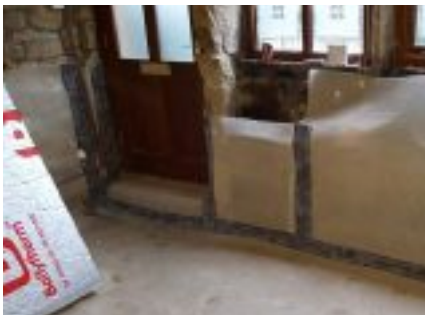
Waterproof membrane during installation.
