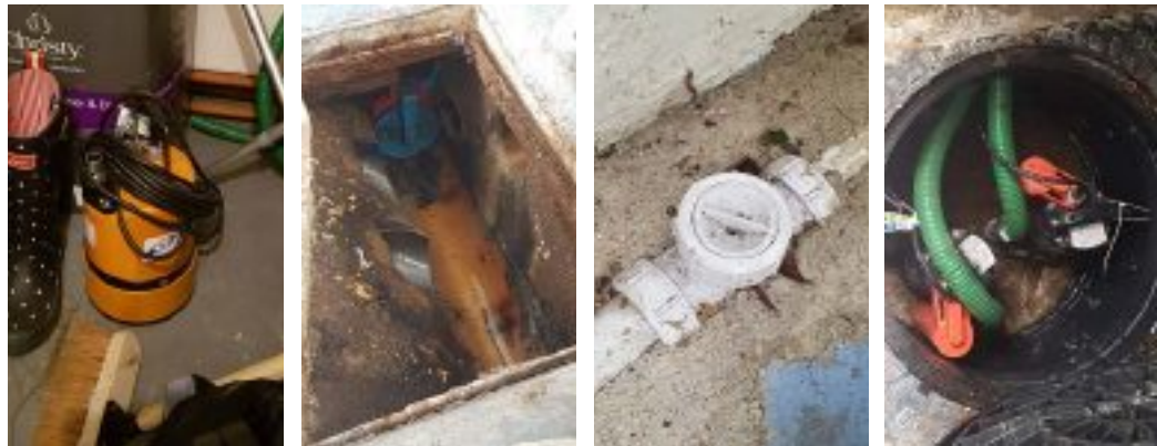
Puddle sucker, non return valves added to all the pipe work and sump pumps in the outhouse.
