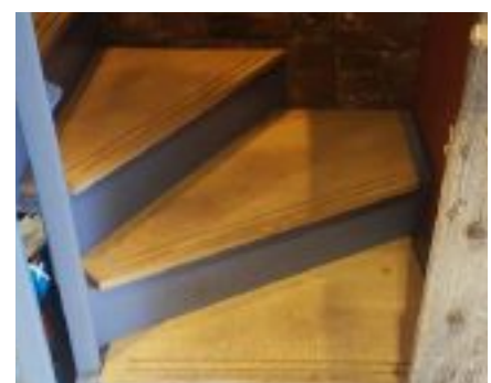
Steel staircase and solid oak treads.
