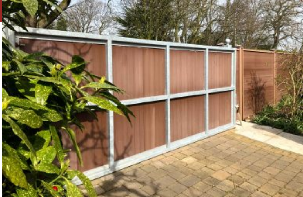
The front entrance gate is the same material as the fence panels and is fitted tightly to prevent ingress of water.
