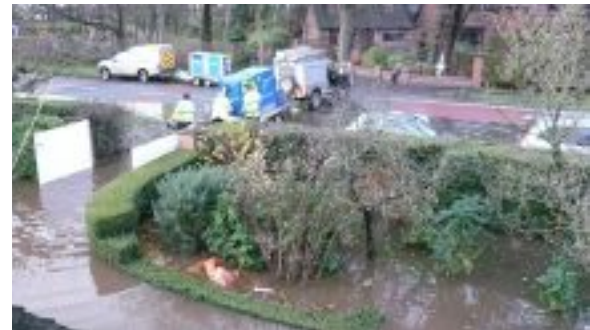
The front entrance gate is the same material as the fence panels and is fitted tightly to prevent ingress of water.
