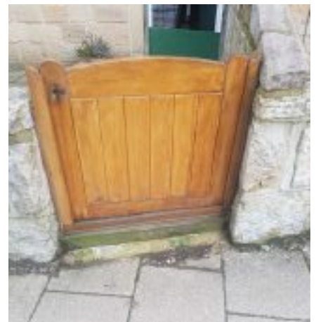
New wall at front of house with a flood-proof gate
