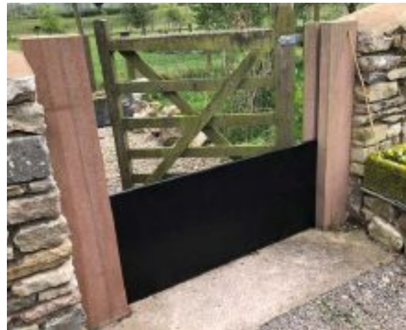
Marine ply slot-in barriers put behind the gates in the wall.
