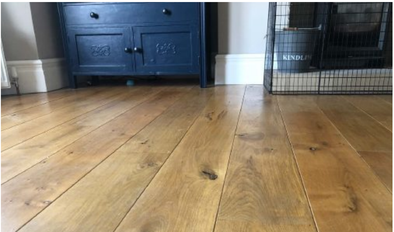
Hard wood flooring with rugs replace the carpets which were a nightmare to lift out and dry following the flood.
