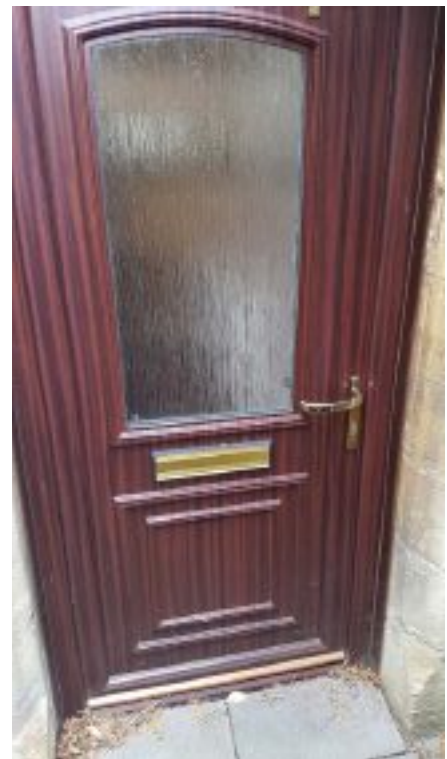
A flood resilient door to the front of the property.
