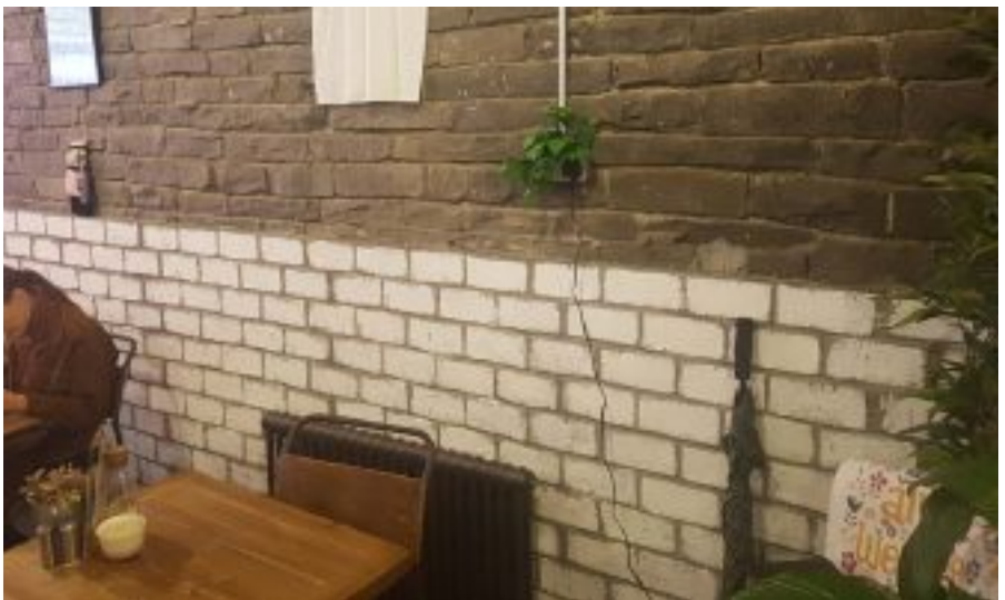
Walls stencilled and painted to resemble tiling.
