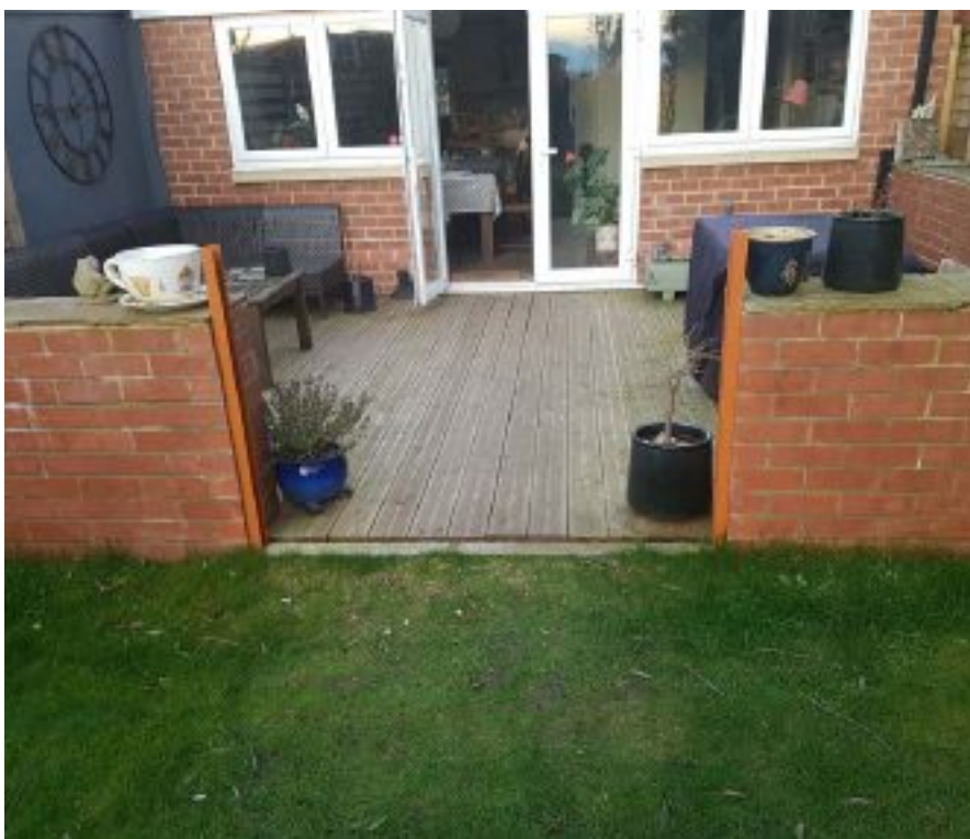
A flood wall has a flood-proof gate for access to the patio area.
