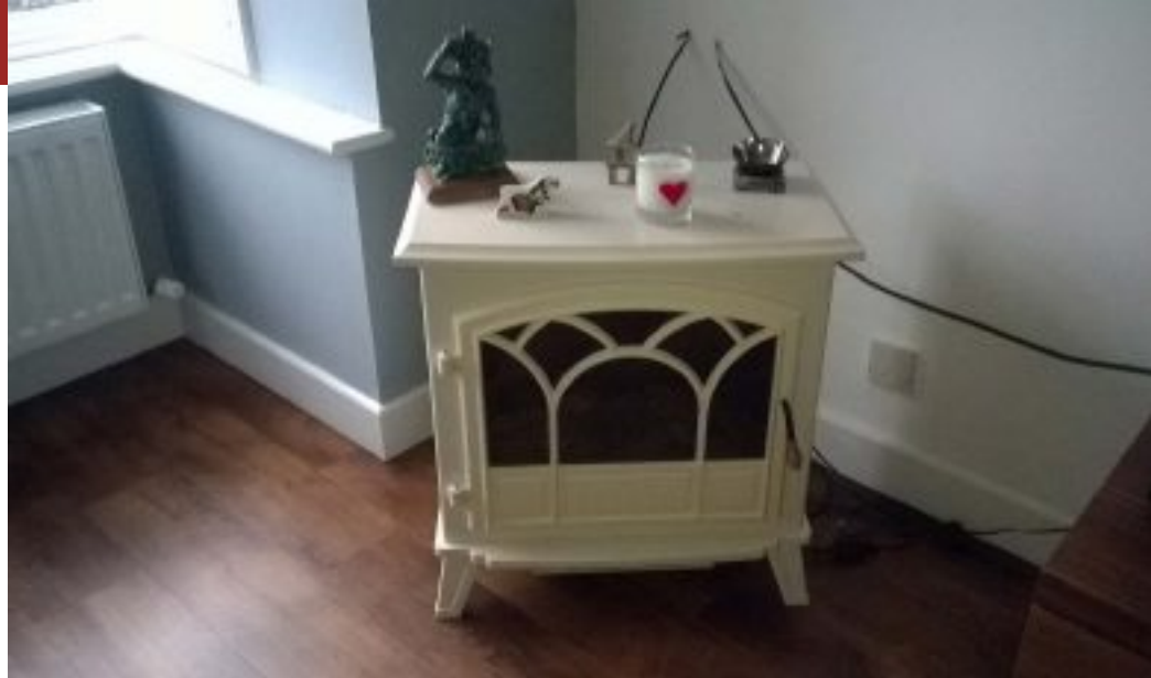
Fires attached to the wall were replaced in all rooms with mobile fires that can be lifted at short notice.
