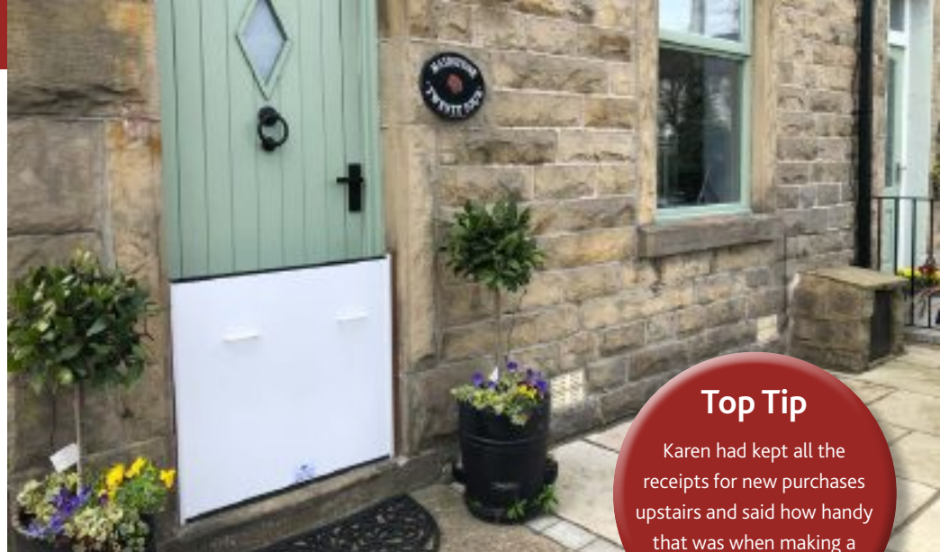
Flood Barrier to basement door and window.
