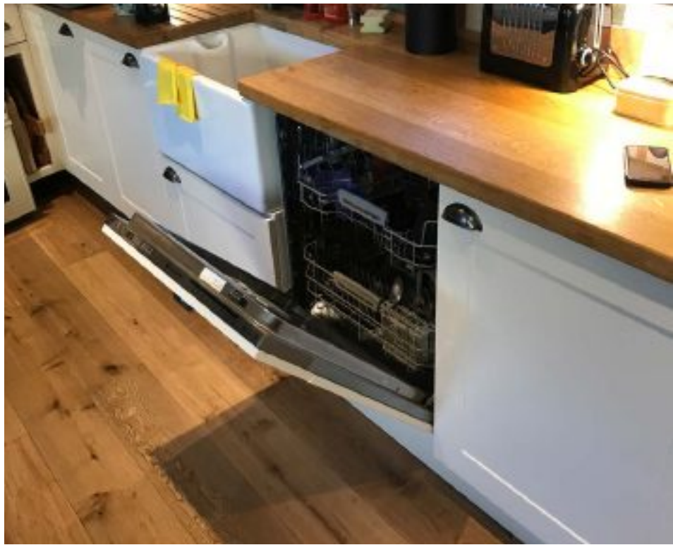
Existing kitchen and floor finishes were removed, and then re-installed following completion of the work.
