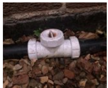
Non-return valve in pipework, to prevent backflow.
