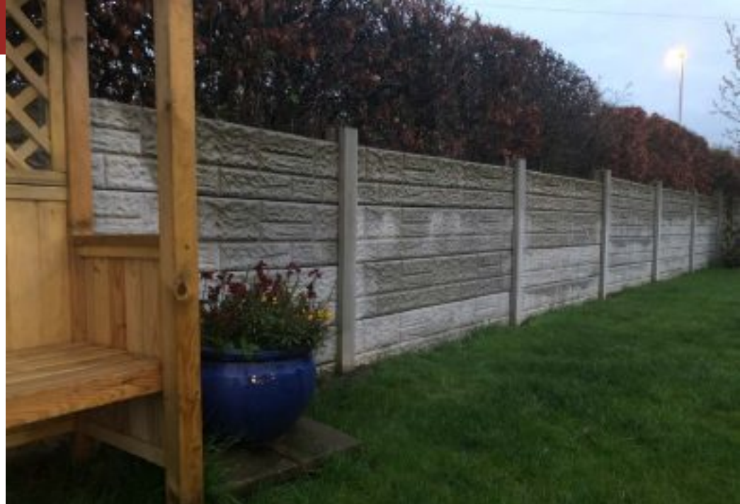
A 'concrete type' fence has been erected to hopefully slow the flow of water, providing extra time to evacuate.
