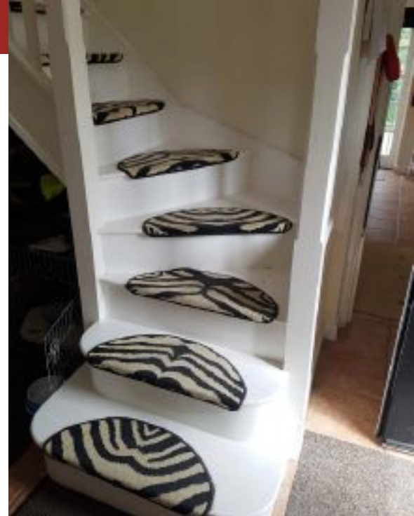
The staircase has only minimal carpet, which can easily be replaced.
