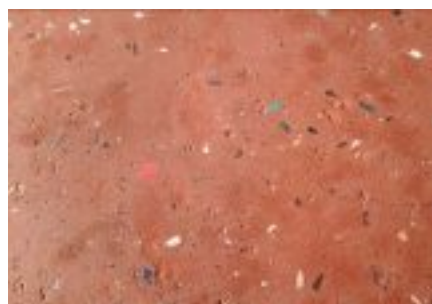
The walls were rendered using coloured renders.
