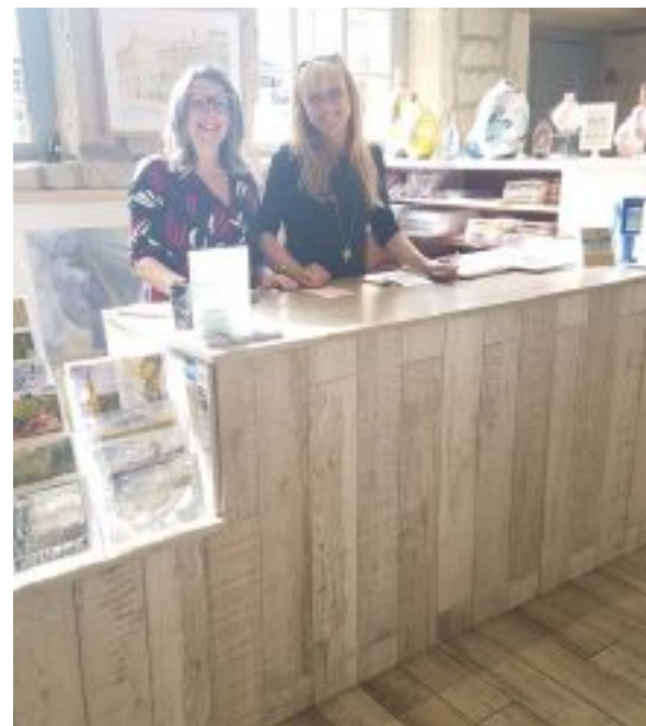
Counter base and new shelving is made from marine ply and coated with sealant.
