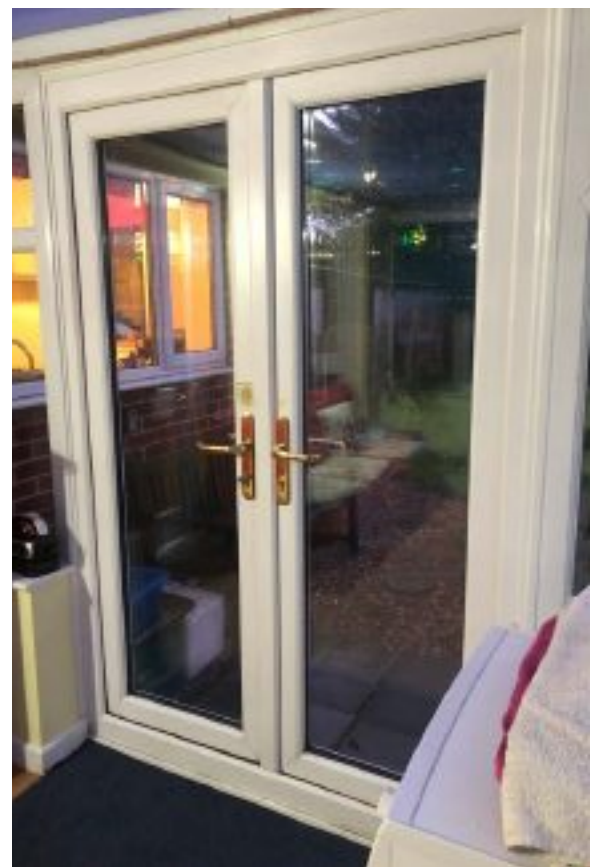
Flood resilient patio doors have been installed.
