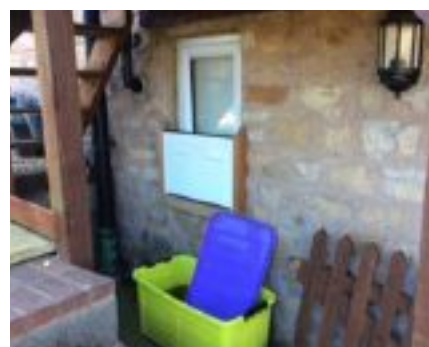
Flood barrier to basement door and window.
