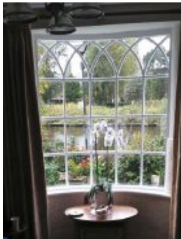
Original Georgian window now reinforced with concrete, and has bespoke barriers.
