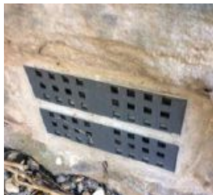
Self-closing airbricks.
