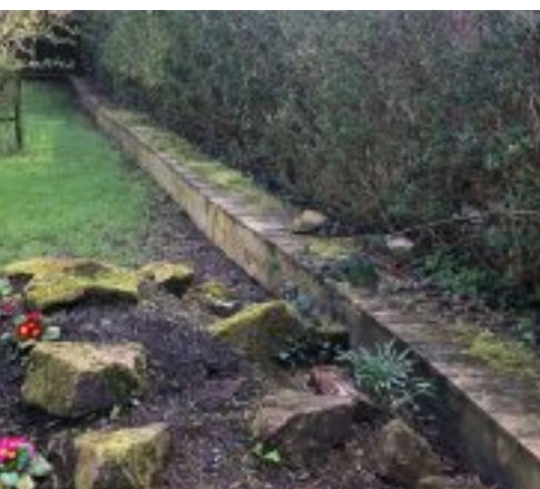
Wall with substantial foundations in the garden.
