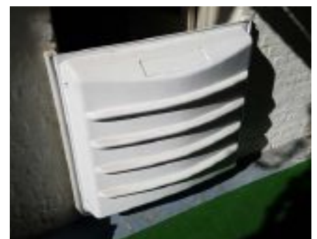
Flood barrier on the back door.
