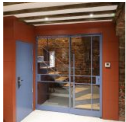
Glazed sliding door/screen in powder-coated steel.
