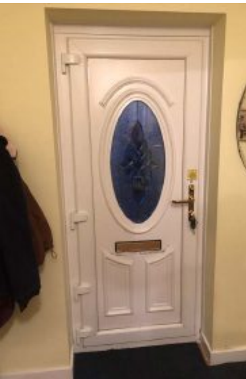
Flood resilient front door has been installed.
