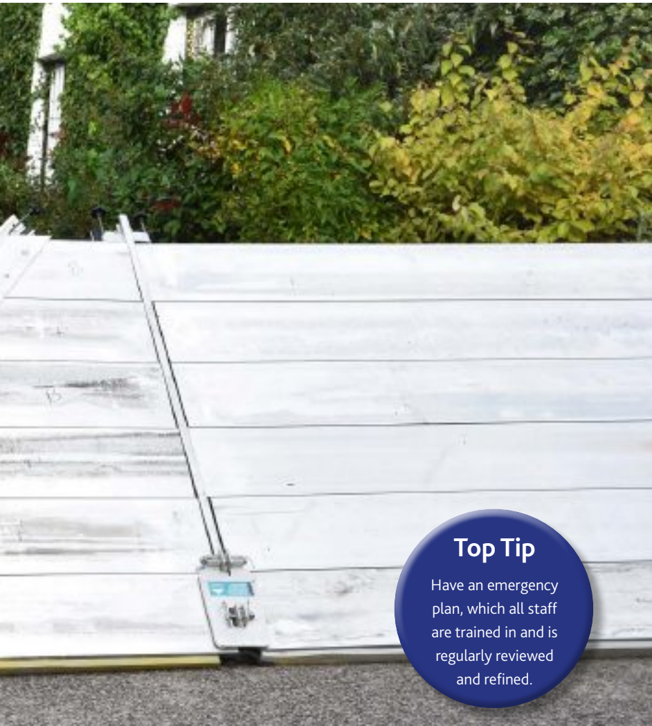
Rigid temporary barriers are installed around the hotel to a height of 1.2m (4'). The hotel has 'Flood Marshals' trained to put the barriers in place, which take 6 people about 1.5 hours.
